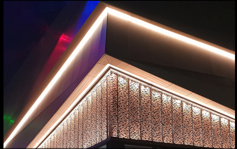
Intu Lakeside Shopping Centre. Lighting design by Hoare Lea
