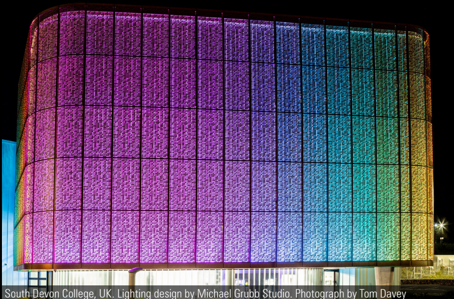
South Devon College, UK. Lighting design by Michael Grubb Studio. Photograph by Tom Davey
